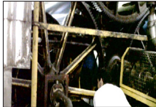
715 Spraflex Gold was applied by a conventional pneumatic grease pump.
